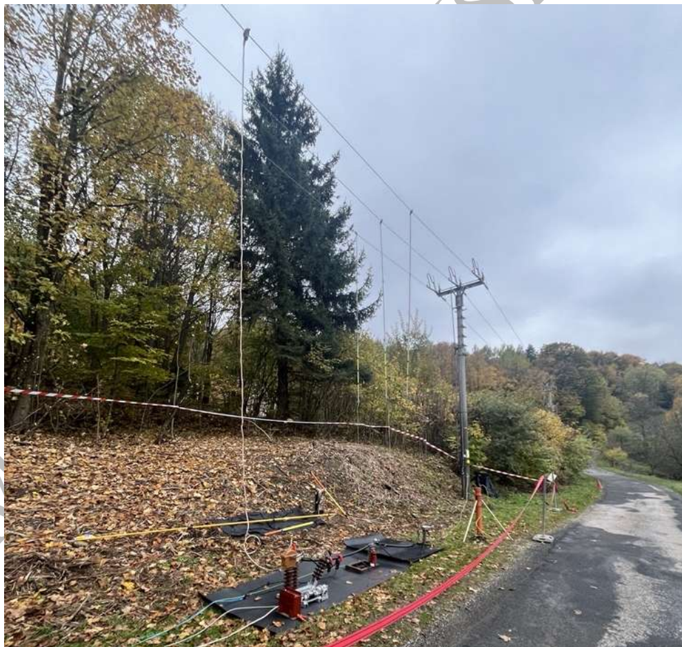
Giant. 2-1 Ground connection at DTS Vlčí 400953
